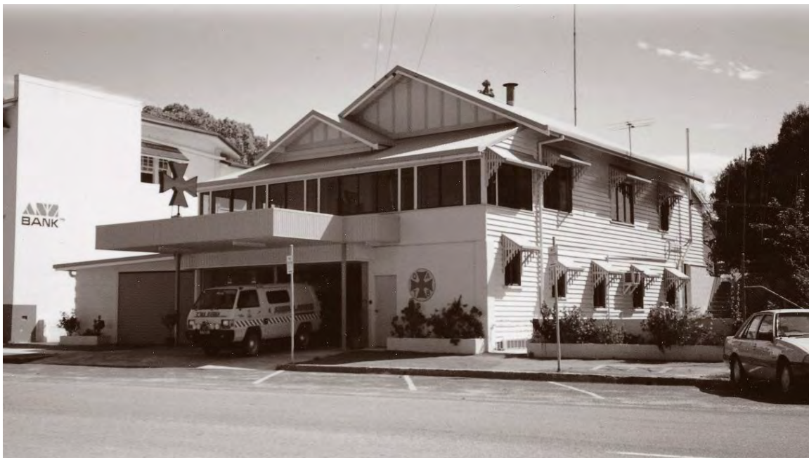
Pomona Sub-Centre building
